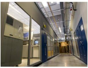
This system is available in both non-fire and fire rated versions to BS476:Part 22: 1987. As well as offering the option of noise reduction capability of up to 32dB. All panels are supplied with a TGIC and lead free powder coat finish which enables a clean and fast install.
